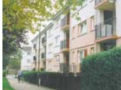
Refurbished flats, Whitburn 1998
